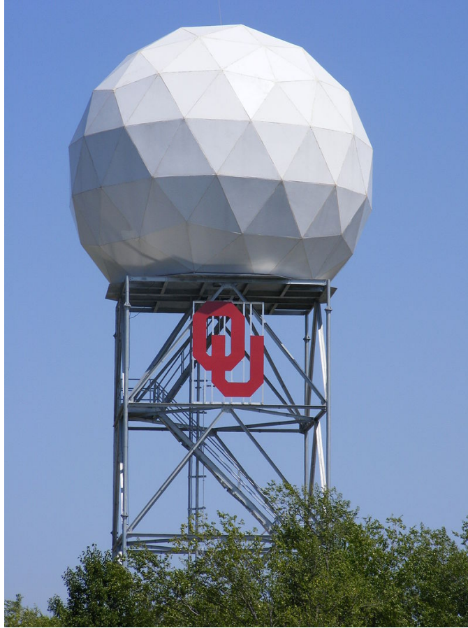
Figure 2.5: The S-band OU-PRIME space-frame radome. The radome stackup is A-sandwich type. Photo source: https://en.wikipedia.org/wiki/OU-PRIME .
